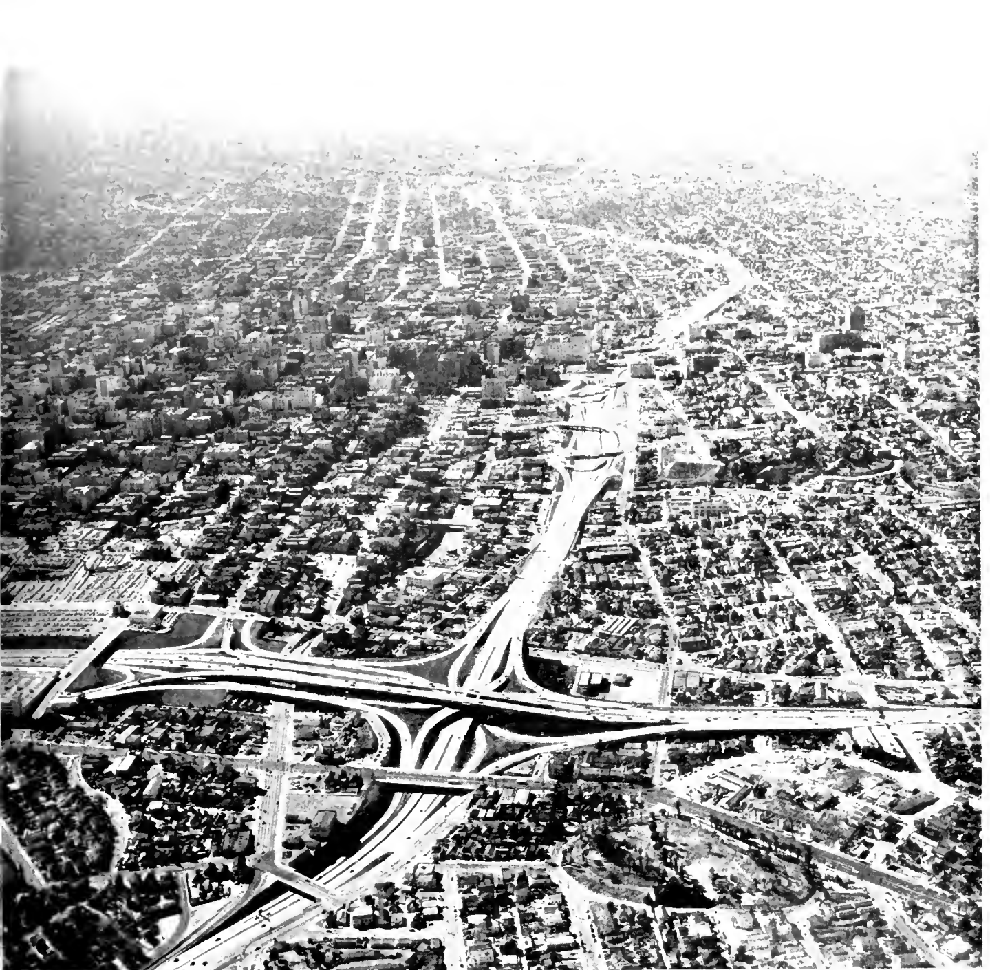
Looking southerly along Harbor Freeway. Four-level traffic interchange shown in center foreground.
